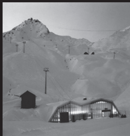
Bearth & Deplazes: Carmenna-Sesslenban, Talstation.
